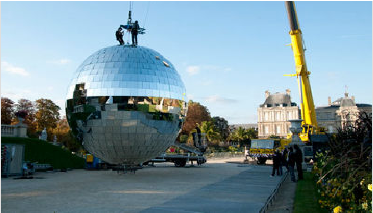
Preparing for lifting.
